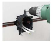
Insert cable on rear side of adapter, fix adapter to the wall.
