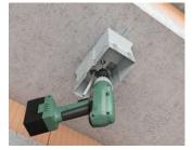
Screw installation housing to the ceiling.
