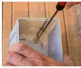
Screw the housing base to the wall.
