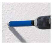
Create installation openings of Ø 20 mm (e.g. KAISER hardened metal cutter with depth stop)
