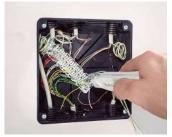
Space for installation of LSA+ terminals for distribution of telecommunication equipment.
