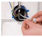
Connect functional earth of the box to tracer wires of screened cable.
