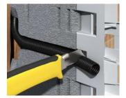
Press the conduit into the side guide and cut it to length.
