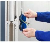
The sound insulation box is simply fixed with plaster.
