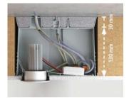
Installation depth 130 mm (insulation thickness 160 mm).
