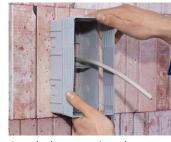
Attach the extension element and snap it into place.
