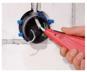
Remove cable sheath and screen with AMZ 2 (Art. No. 1190-02). Fit bare tracer wire with transparent insulating hose.
