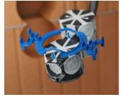
Position the KLEMMFIX® on the bottom of the box...
