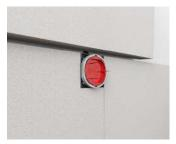
Apply the internal insulation around the box.
