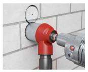
Fit diamond grinding head and diamond cut Ø 68 mm or Ø 82 mm holes.
