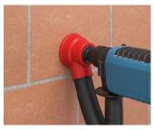
Cut a Ø 82 mm installation opening using a grinding head (e.g. Art. No. 1088-02).
