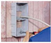
Screw the housing base to the wall.
