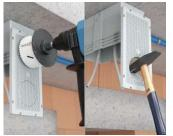
Ceiling exit ø 68 mm for knocking in, ceiling outlet up to ø 86 mm for cutting out.
