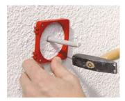
If a cable is present, you can drill 68 mm installation openings using the hardened metal cutter 180.
