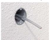
Flush-mounting and secure fit of the one-gang box.
