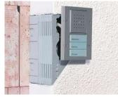
After applying the plaster, attach the desired accessory.
