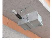
Break out the conduit entry or cut an exact cable entry for airtight installation, e.g. by using the KAISER universal opening cutter (Art. No. 1085-80).
