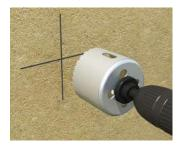
Cut the Ø 68 mm installation opening using a suitable cutter (e. g. Art. No. 1083-70; countersink hole cutter and ejector spring must beremoved).
