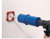
Using carbide cutter 180 (Art. No. 1088-07), cut the installation opening precisely as far as the depth stop.
