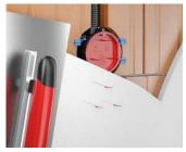
The fine marker bristles of the signal cover indicate the exact position of the one-gang box after plastering.
