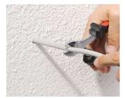
Ensure that the cable was fed through the insulation material panel. Shorten the existing cable to approximately 10 cm.
