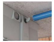
Insert the conduit or cable into the installation housing; fit sealing plug to the conduit.
