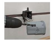
Cut exact and air-tight cable entry using a drill.
