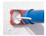
Using the combined cutting aids (Art. No. 1090-68), cut installation openings at the standard spacing of 71 mm.
