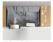
Installation depth 100 mm (insulation thickness 130 mm).
