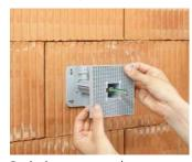
Push the one-gang box onto the supporting arm as far as the stop.
