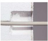
The depth stop ensures minimal interference with the insulation, which prevents the creation of heat bridges.
