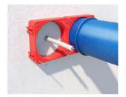
Using cutter (Art. No. 1088-07) and two centering aids (Art. No. 1090-68), cut two installation openings at least 55 mm deep and with a diameter of 68 mm
