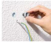
Press the anchor sleeve of the mini equipment carrier into the installation opening so that it is flush with the wall.
