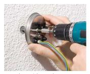
...and provide a tolerance compensation of up to 10 mm. This permits later exact alignment of all installation accessories.
