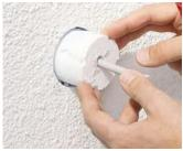
Remove the drilled core from the opening.
