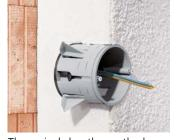
The swivel sheaths on the box seat themselves securely in the insulation material.
