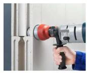
Cut a Ø 82 mm installation opening using a grinding head (e.g. Art. No. 1088-02).
