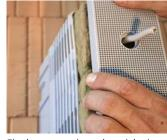
Fit the mounting plate (closing clip underneath) and close.
