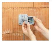
Push the one-gang box onto the supporting arm as far as the stop.
