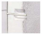
The opening is now only as deep as necessary. The insulation remains intact and the cable is undamaged.
