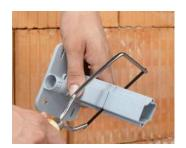
Saw the carrier to the required length. The integrated indicated dimension ensures exact reading of the dimension.
