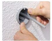
Press the box in the holding ring until the rim is flush with the wall.
