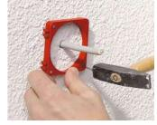
Fasten the KAISER centering aid Ø 68 mm (Art. No. 1090-68) to the composite thermal insulation system using steel nails.
