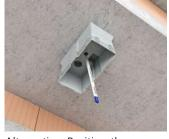
Alternative: Position the installation housing with the alignment markings for the luminaire and mark the drill hole.
