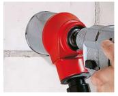
Cut an accurate wall opening (Ø 82 mm) with the diamond grinding head.
