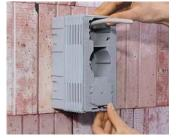
Position the combination insert (mounting clip at bottom) and snap into place.
