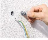
Press in the attachment core until it locks into the anchor sleeve.
