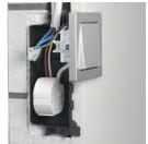
Here for example is a relay for central control of several roller blind drives or a flush mounting EIB interface with a conventional button.
