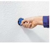
The ECON® Iso + or Styro55 with the swivel cutters are mounted quickly and easily with the setting tool.
