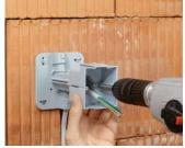
The front fixing and the depth stop always ensure exact fitting and prevent incorrect installa-
