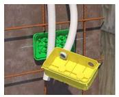
Insertion of the conduits through exact openings.
