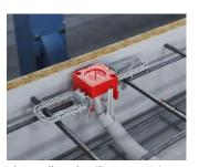
The wall and ceiling transitions are pre-fixed in the reinforcement using Prefix® installation technology and fixed with tie wires, then the conduit connection is made.
