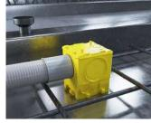
Clip the conduit connector into place and insert the conduit into the conduit connector.
