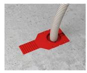
Insert the conduit into the clean installation opening.
