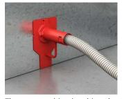
The exact position is achieved with the help of the measurement strip and by gluing it to the formwork edging.
