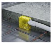
The system magnet is used to hold B<sup>2</sup> one-gang junction boxes,
