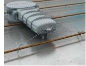
Alternatively, tie lugs fitted at the end of the tunnel provide additional protection against the possible floating of the tunnel in precast concrete.
