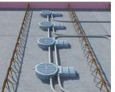
After fitting of the conduits, concreting on the planned ceiling thickness takes place with the on-site mixed concrete process.
