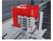
The required concrete ceiling can be quickly read off and precisely set using the dimensional scale. The dimensional scale is adjusted, so that the wall-ceiling transitions are minimally below the subsequent wall surface,
