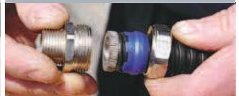
Bring the body to mate with the back nut. Metal fittings should be tightened with grips or spanner to ensure security and IP rating.
