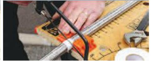
Cutting of overbraided conduit is made much easier by tightly wrapping self adhesive tape around the conduit and sawing through the middle of the tape. The tape should be removed after cutting if EMC screening is required. Ensure you make a straight vertical cut.
