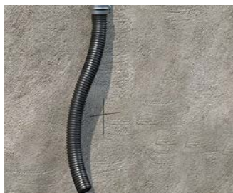
Masonry with conduit exit.
