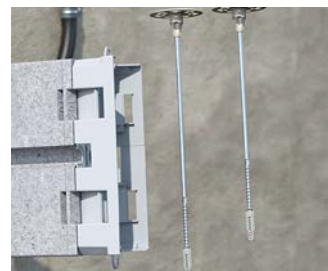
Remove the side lugs from the screw dowel. Note the different lengths!
