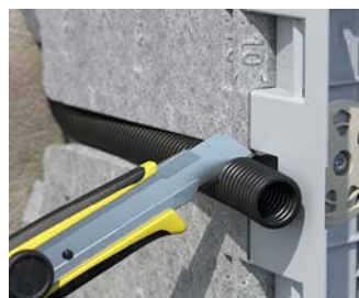
Press the conduit into the sideways guide and cut it to length.
