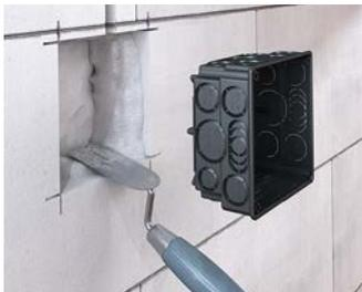
Make an appropriate wall opening, feed the cables and conduits into the housing and fasten it (using plaster) in the wall.
