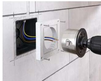
You can create the installation opening before or after inserting the housing. The equipment is attached by simply clamping it in or screwing it into the mineral fibreboard.
