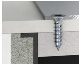
Use only screws that go into but not through the mineral fibreboard when attaching the device! (e.g. SPAX countersunk head screw 3.5 x 15 mm)!
