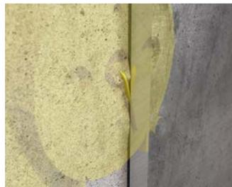
The signal bristle on the front parts of the Flat 45 system boxes clings to the formwork when it moves and keeps its position visible in the wall surface.
