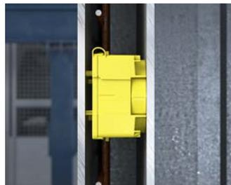
The slots on the back of the Flat 45 system boxes are used in 50 mm walls to support the back of the box against the formwork and prevent the box from tilting when fixed on the back.
