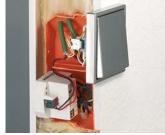
The electronics box offers a generous installation space for the decentralised installation of small window actuators for controlling blinds and heating, for example.
