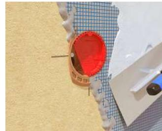
Before plastering, fit the signal cover (Art. No. 1181-60). Protects the interior of the box, the screw domes and the screw heads.
