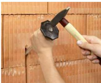
Prepare the cable routes. Try to avoid direct cable routing through masonry and insulation.
