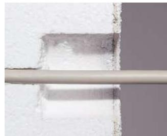
The depth stop ensures minimal interference with the insulation, which prevents the creation of heat bridges.
