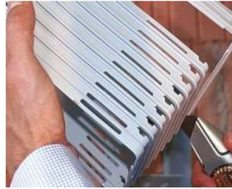
If necessary, adjust the extension element to suit the insulation thickness.
