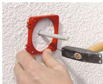
Fasten the KAISER centering aid Ø 68 mm (Art. No. 1090-68) to the composite thermal insulation system using steel nails.
