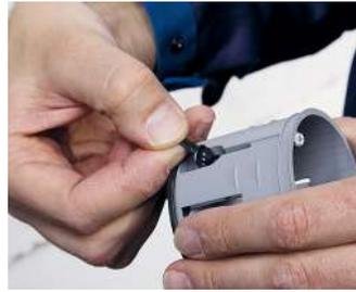
Before inserting the support connector, remove the strap without using a tool.
