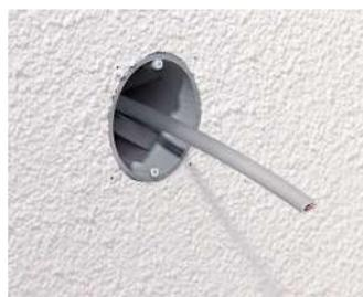
Flush-mounting and secure fit of the one-gang box.
