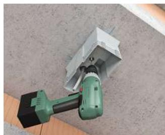
Screw installation housing to the ceiling.
