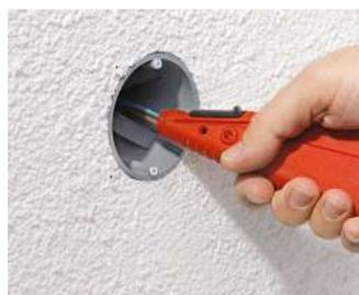
Using the KAISER stripping pliers, (Art. No. 1190-02), remove the insulation from the cable.
