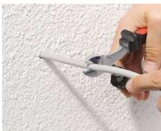
Ensure that the cable was fed through the insulation material panel. Shorten the existing cable to approximately 10 cm.
