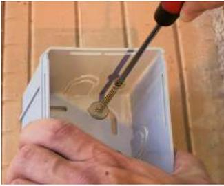
Screw the housing base to the wall.
