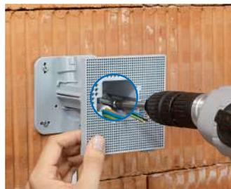
The front fixing and the depth stop always ensure exact fitting and prevent incorrect installation.
