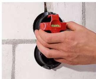
Push the box combination into the wall opening and align.
