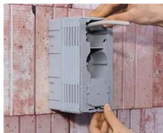
Position the combination insert (mounting clip at bottom) and snap into place.
