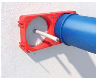
Using cutter (Art. No. 1088-07) and two centering aids (Art. No. 1090-68), cut two installation openings at least 55 mm deep and with a diameter of 68 mm.
