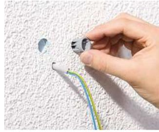
Press the anchor sleeve of the mini equipment carrier into the installation opening so that it is flush with the wall.
