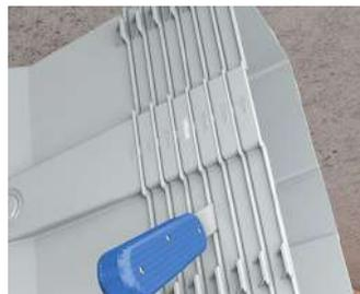
Adapt installation housing to the insulation thickness.
