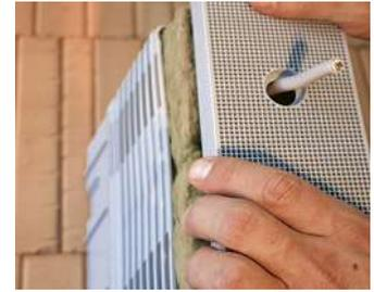
Fit the mounting plate (closing clip underneath) and close.
