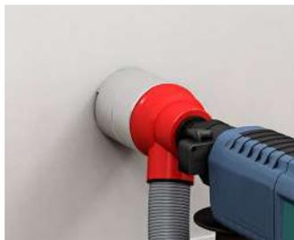
For insulation thicknesses < 100mm, cut wall opening (Ø 82mm).
