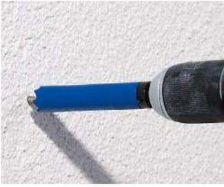
Create installation openings of Ø 20 mm (e.g. KAISER hardened metal cutter with depth stop).
