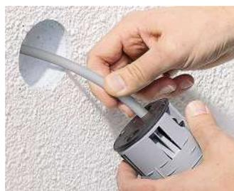
The ECON® technology elastic sealing membrane ensures a wind-tight seal around the cable as it is pushed through.
