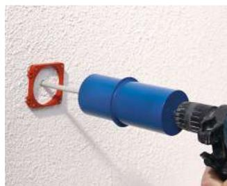
Using carbide cutter 180 (Art. No. 1088-07), cut the installation opening precisely as far as the depth stop.
