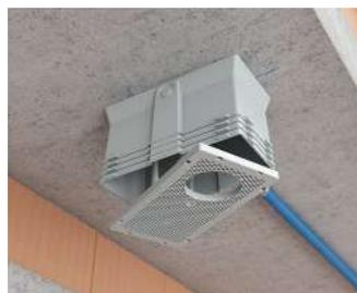
Depending on the required installation diameter ceiling exit of  $\varnothing 68$  mm or up to  $\varnothing 86$  mm, turn the front part by  $180^\circ$  and latch into Position.
