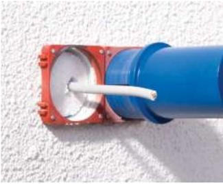
Using the combined cutting aids (Art. No. 1090-68), cut installation openings at the standard spacing of 71 mm.
