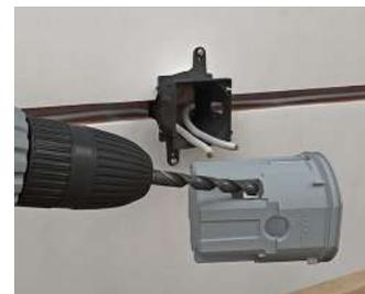
Cut exact and air-tight cable entry using a drill.
