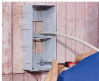
Screw the housing base to the wall.
