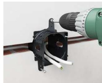
Insert cable on rear side of adapter, fix adapter to the wall.
