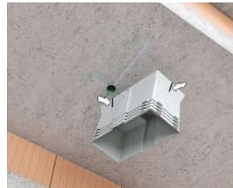
Alignment markings for the luminaire position and the fixing point.
