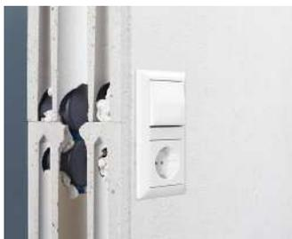
Example of installation using a switch-socket combination.
