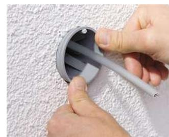
Press the box in the holding ring until the rim is flush with the wall.
