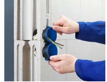
The sound insulation box is simply fixed with plaster.
