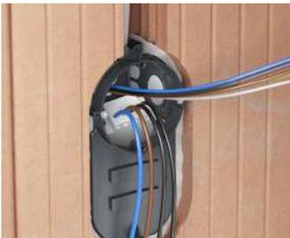
By inserting the separator wall, two different voltage types can be fitted in a standardised way in the electronics box. In addition, they provide a generously-sized installation space...
