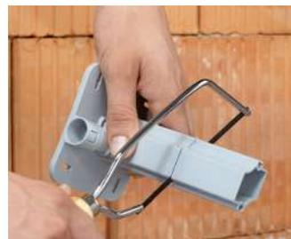
Saw the carrier to the required length. The integrated indicated dimension ensures exact reading of the dimension.
