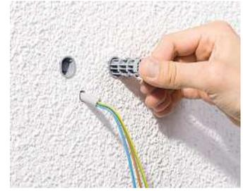
Press in the attachment core until it locks into the anchor sleeve.
