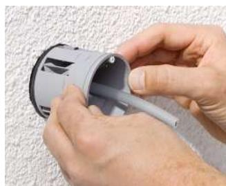
Simply insert the ECON® Styro55 one-gang junction box in the installation opening.
