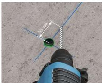
Drill a  $\varnothing 8$  mm hole for a standard dowel and insert the dowel.
