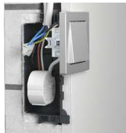
Here for example is a relay for central control of several roller blind drives or a flush mounting EIB interface with a conventional button.
