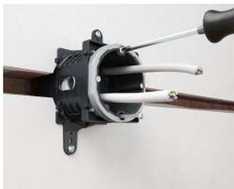
Insert cables into box, screw box to Adapter.
