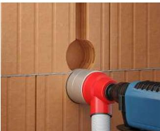
Make the installation opening  $\varnothing 82$  mm with the diamond grinding crown (Art. No. 1088-02).
