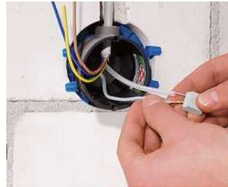
Connect functional earth of the box to tracer wires of screened cable.
