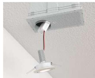
Applying insulation and plaster. Fitting the LED installation spotlight with plenty of space for the ballast device.
