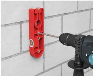
Pre-drilling. Create centering hole at a combination distance for multiple boxes using drilling template.
