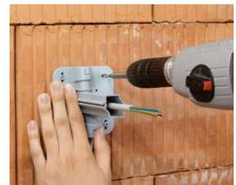
Slotted holes allow precise alignment even when the drill holes are not exact.
