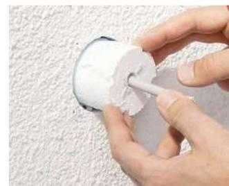
Remove the drilled core from the opening.
