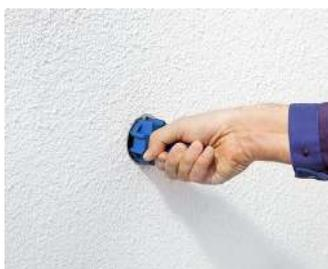
Use KAISER tool (Art. No. 1090-22) to position the four swivels in the catch mechanism.
