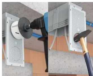
Ceiling exit  $\varnothing 68$  mm for knocking in, ceiling outlet up to  $\varnothing 86$  mm for cutting out.
