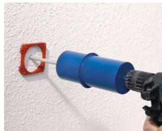
The centering aid Ø 68 mm and depth stop on the cutter ensure a precise opening without damaging the existing cable.
