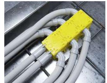
3-unit combination with inserted conduits in the wall area.
