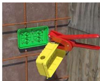
Make conduit entry (punch pliers or universal opening cutter).
