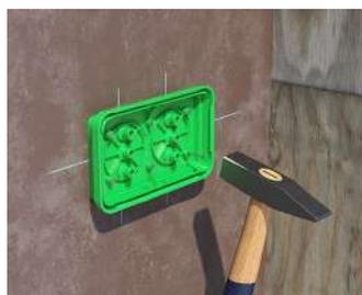
Fix the front part to the formwork (nail or screw fitting).
