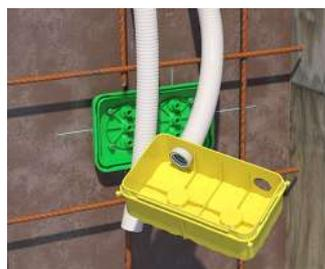
Insertion of the conduits through exact openings.
