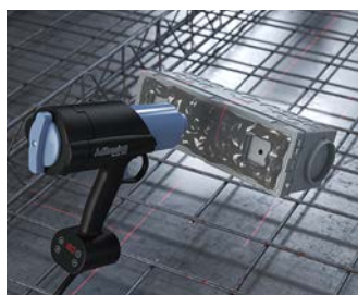
Fixing by means of hot glue.
