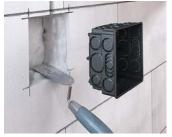
Make an appropriate wall opening, feed the cables and conduits into the housing and fasten it (using plaster) in the wall.
